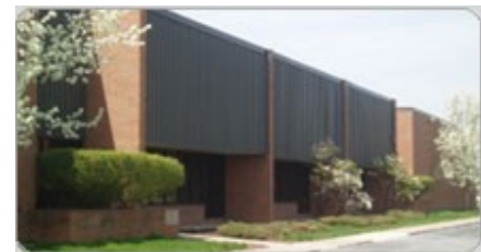
IB opened the first U.S. large prismatic lithium battery plant in 2008
