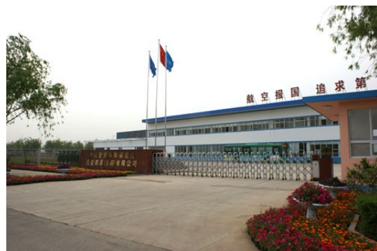
Sky Energy facility, Luolang, Henan
